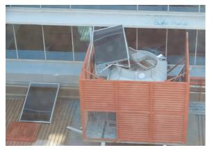
the cause, engaged an engineer to conduct a forensic investigation to determine the contributing factors. The Strata Manger shared the Engineer's Report with AGWA. It indicated that insufficient fixings had been used in securing the window frame and that, together with the excessive wind load on the day, had caused the window to fall.
